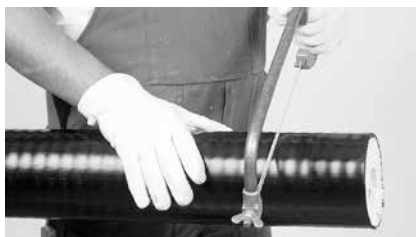
2 Cut the casing pipe with saw.
