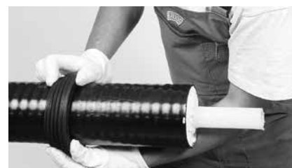
6 Install the wall sealing ring.
